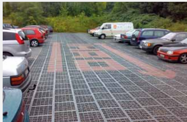
A company car park at Hans Ihro GmbH with the company logo made out of TTE® paving (the ballast is filled flush with the surface).
