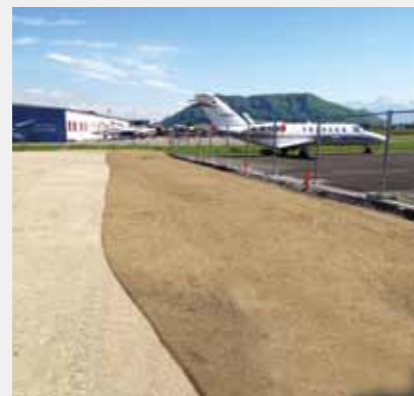
Applying and levelling of the bedding (grit-top soil-mixture)
