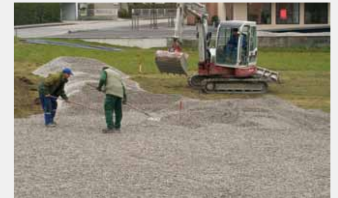
2. Application and skimming of the mineral structural component
