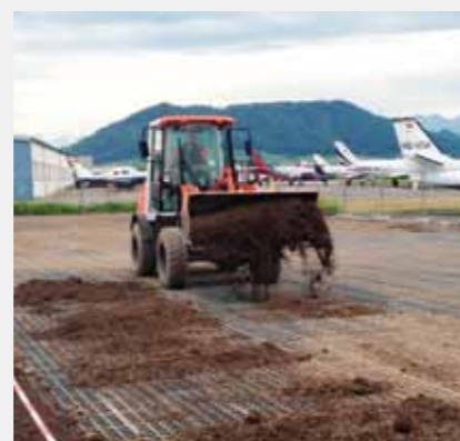
Introduction of the substrate (top soil-sand-mixture) as a chamber filling; seeding and completion
