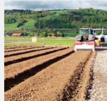
Rolling on the gravel sand into the top soil in the ratio 60 % gravel sand: 40 % top soil
