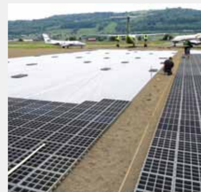
Laying of elements on the fine network as a laying aid and separating mesh
