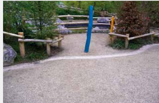
A finished water-bound covering as a pathway reinforcement in the All-weather Zoo in Münster.
