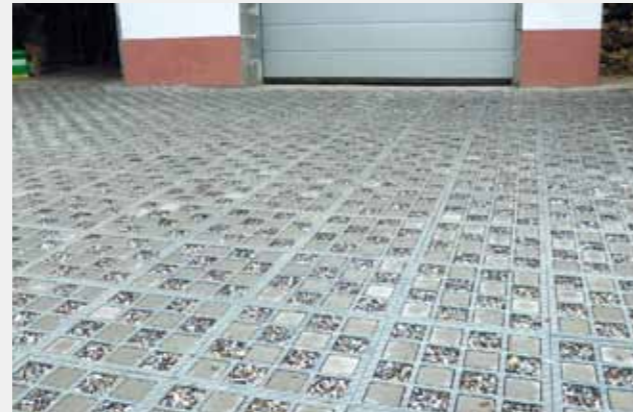
TTE® paving with gravel: permanently loadable, even and permeable
