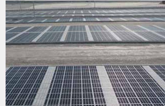
A parking place with a four row parking place marking requires 40 stones per running metre. This allows comfortable loading and unloading. (Mounting during the construction phase)
