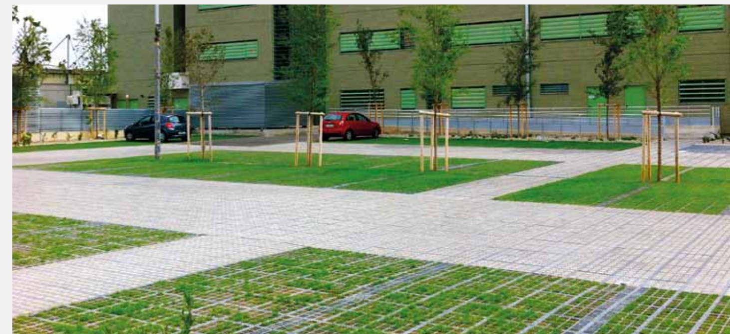
TTE® Construction Principle 2: public parking spaces as TTE® paving stones and TTE® Green (with root protection for tree plantations at the same time)
