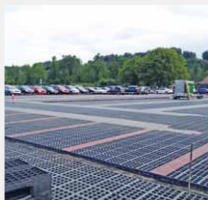
Inserting the TTE® paving stones in the TTE® construction elements as a parking place marking and footpath
