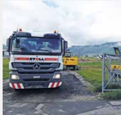
Removal of turf; delivery of gravel base course material
