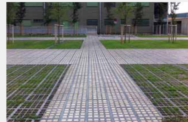
Driving lane and footpath reinforcement with TTE®. Greened and paved areas in an interconnected system.
