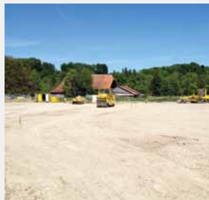
Creation of the terrain modeling and rough grading
