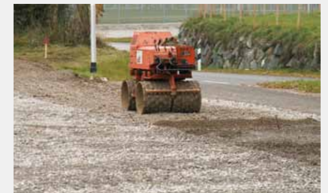
4. Compaction and creation of the planum
