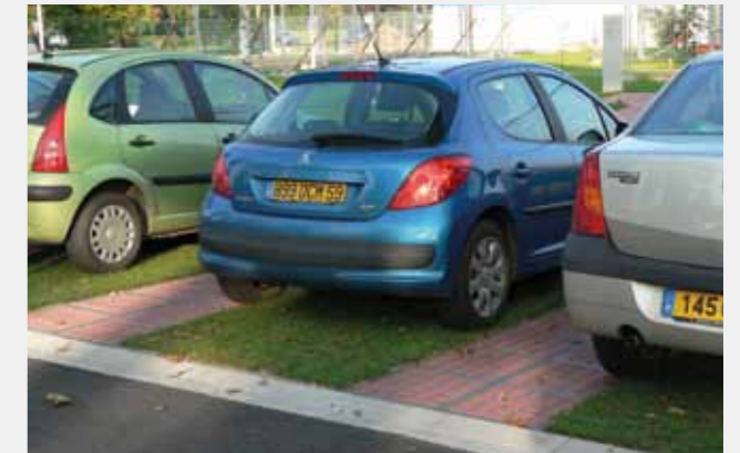
For a wider design of the parking place markings this also, at the same time, offers a reinforced entry and leaving area which can be used under all weather conditions.
